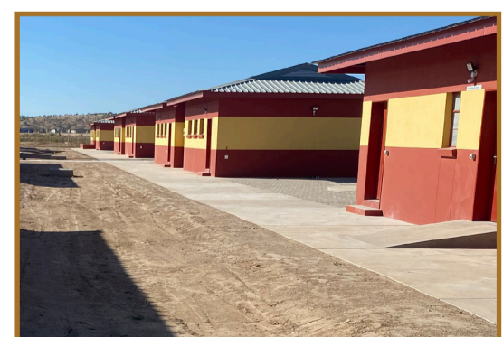
Construction of Otuzemba Primary School
