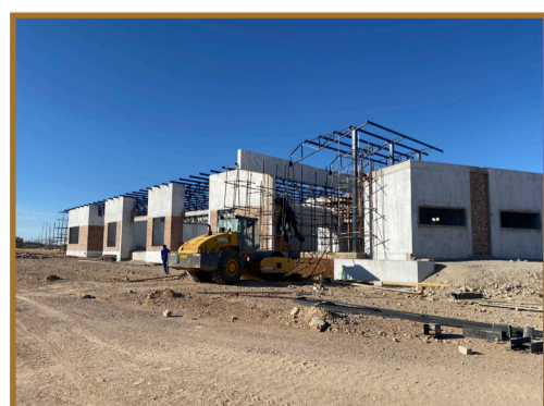
Construction of Kunene VTC
