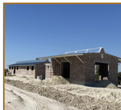
Construction of Station Building: Northern Railway
